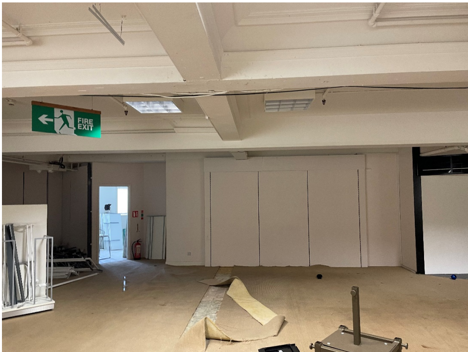
Image of inside the building pre-work being done.
